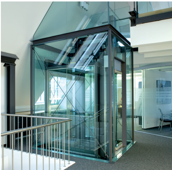
The elevator installed under the roof slope illustrates a custom solution where the xPack delivers clear economic benefits through harmonized components and centralized support.
